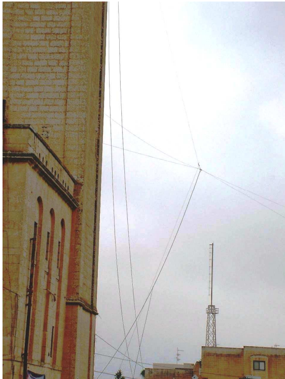
Two dipoles with a common coax feeder
